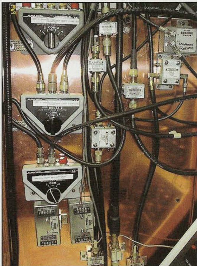
This photo, taken in the author's ham shack, shows a "single point ground" panel with various coax switches that put unused antennas to ground, along with several brands of lightning arrestors. The copper sheet is "bonded" with the outdoor ground system with a 6 inch wide copper strap. The sheet is .022 inch thick copper screwed to a 3/4 inch thick plywood panel.
